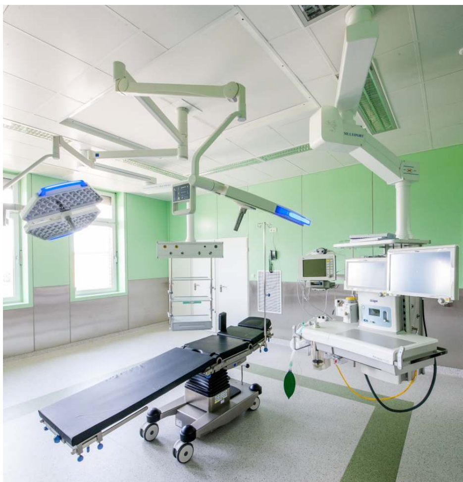
High adjustable ceiling pendant with hanging module for anesthesia machine or other workstations
